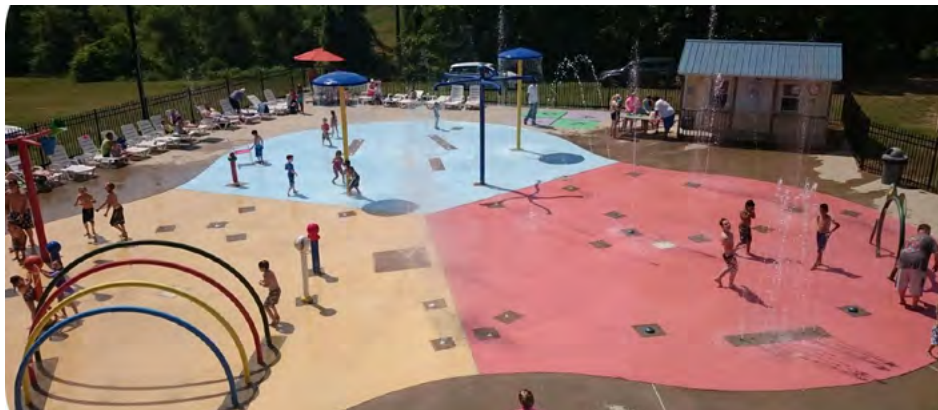
Example of splash pad and full community center (no pool)
