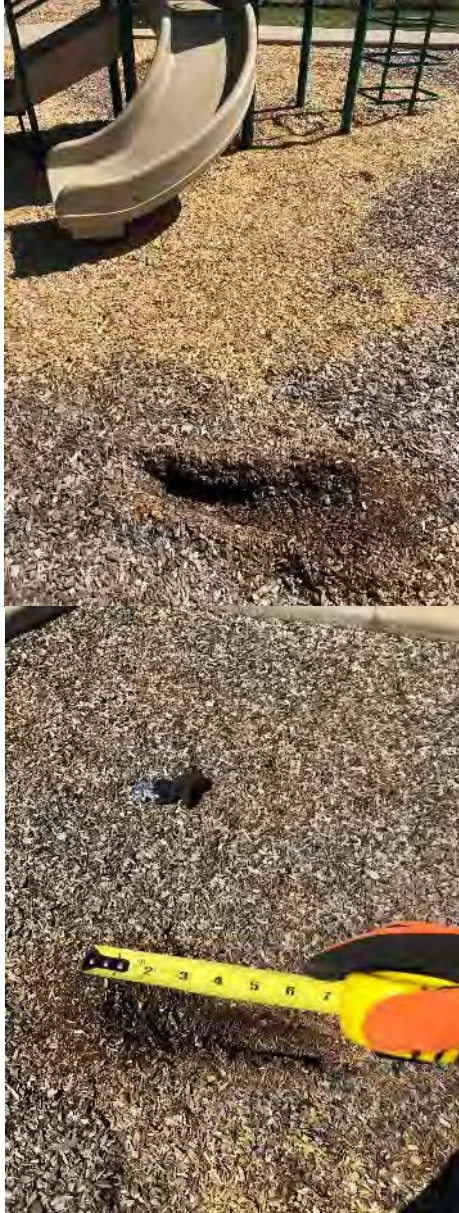
Surface material was 6 inches
