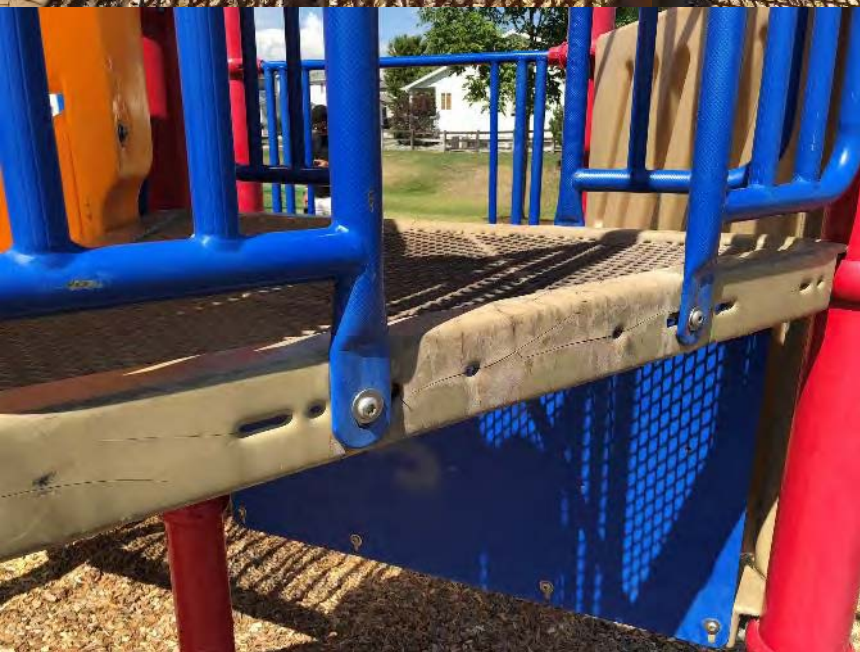
Cracking on the platform
