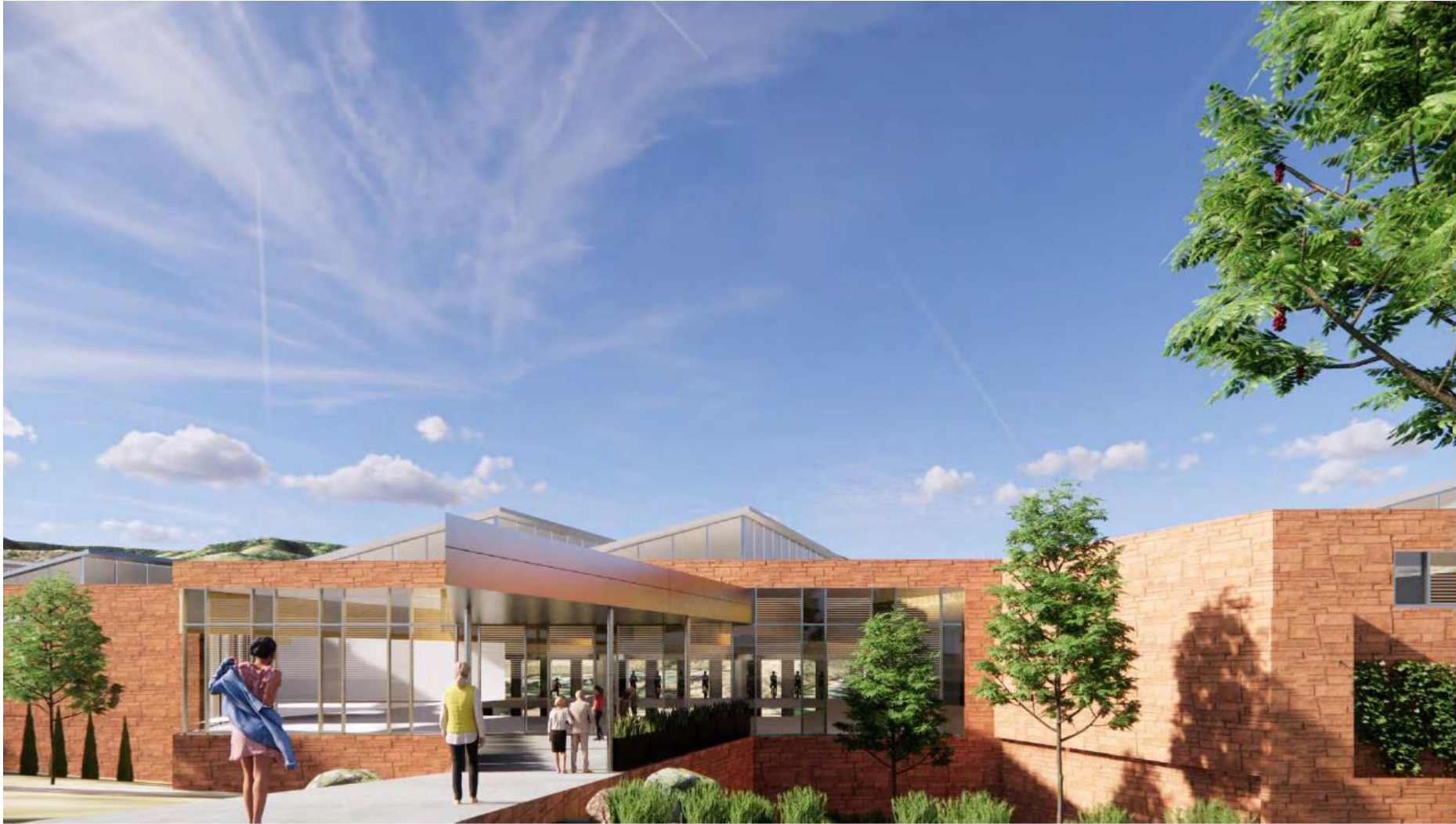
East Side - Entryway -close-in view of covered entryway
